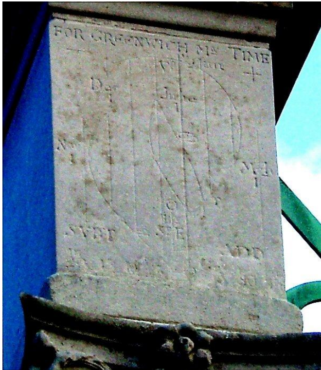
Fig. 14. The EoT graph on the west side of the Abbey Gardens, Bury St Edmunds, pillar dial.
