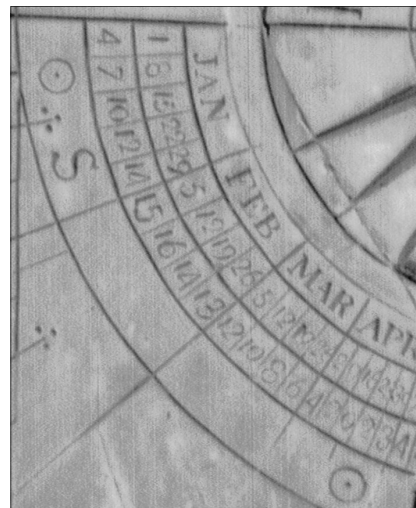
Fig. 8a (above): Camborne church dial, Cornwall. Fig. 8b (left): close-up of the EoT scale. Photos: L. Burge.
